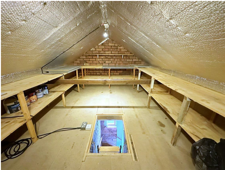
The loft is boarded with shelving, power and lighting.
